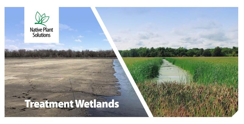
Treatment wetlands are human-made, engineered systems that use natural wetland elements like plants, algae, microbes, light, water and soils to improve water quality. The benefit of these systems is that they can provide high-efficiency water quality treatment with very low operator input.
